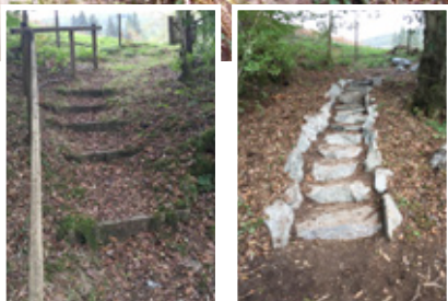
Lauder site access before and after path building work
