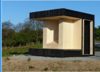
Newly completed Scottish Scenic Routes Structure (SSRS) named 'Gaels View' © RSPB
