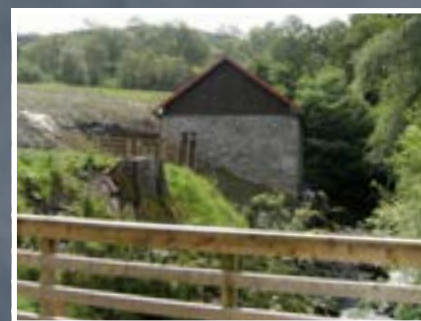
Ardvorlich turbine house
