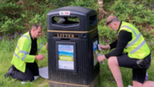
Installing bin sponsor posters
